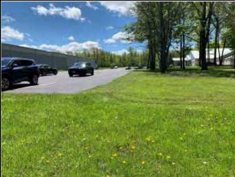
Photo-35 From the area between the stormwater basin and existing substation on City of Amherst property towards the parking lot and southeastern end of Project area
