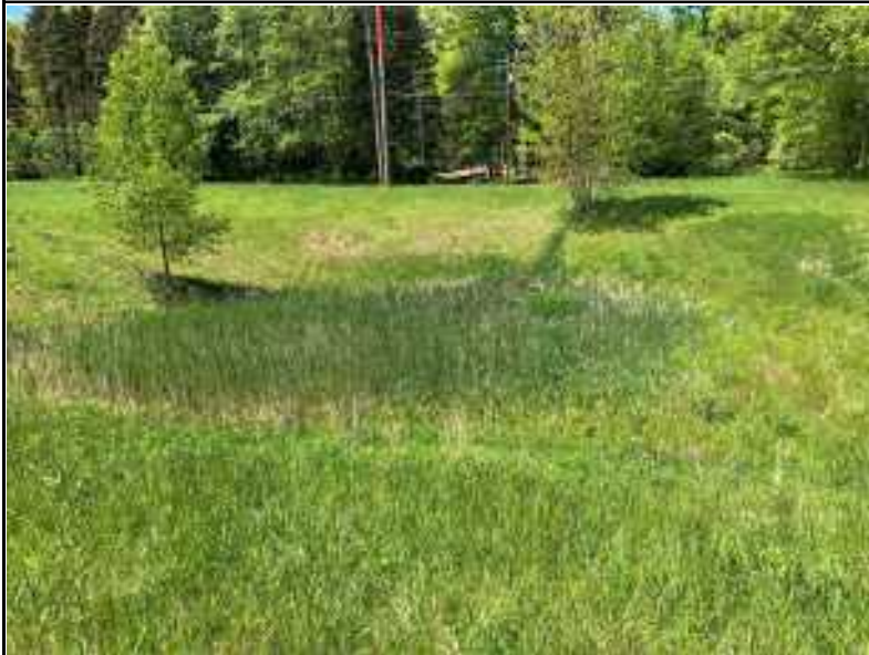
Photo-32 From the area between the stormwater basin and existing substation on City of Amherst property towards stormwater basin
