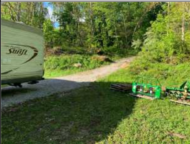
Photo-3 From western end of Project towards quarried landform and access road to existing tline on ROW
