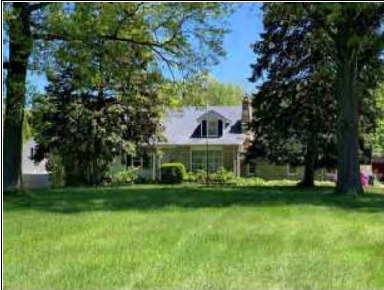
Photo-56 Elevation of Resource B-02 on Cross Road Direction: East Date: 05/13/21 Photographer: Liz Sefton
