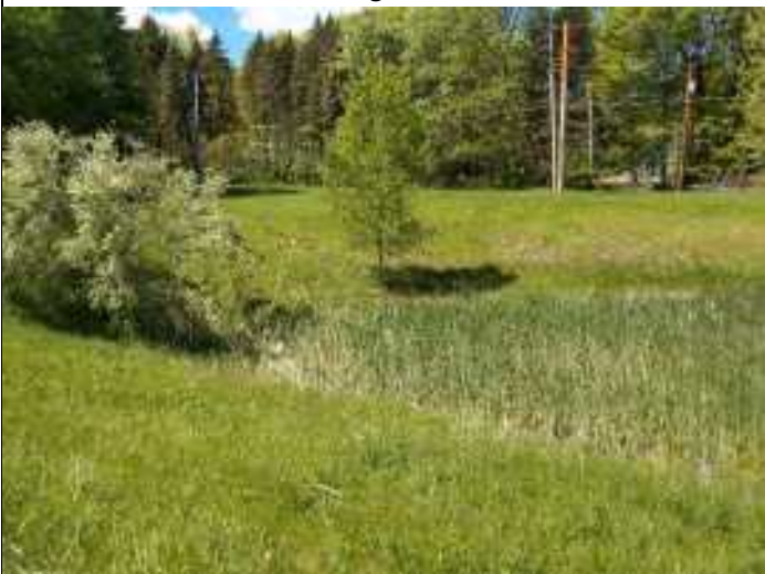
Overview of stormwater basin near UDP-A facing Southwest
