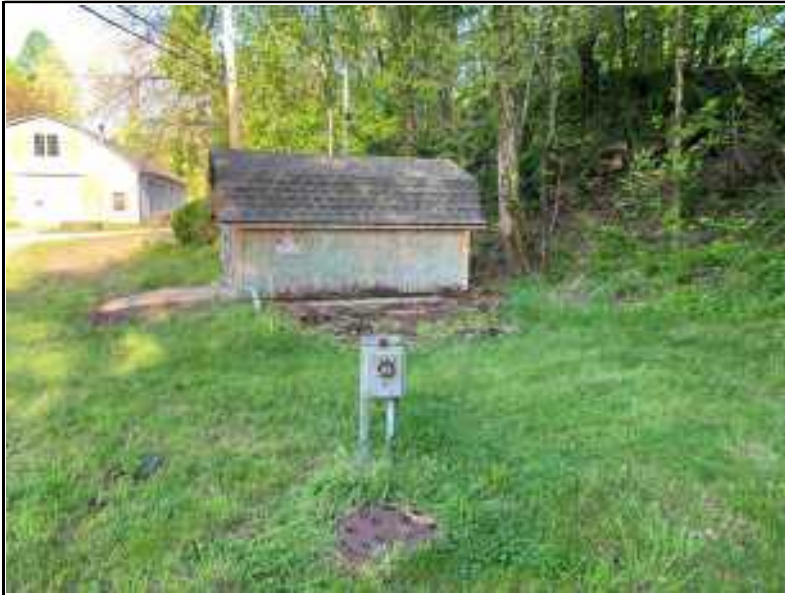
Photo-4 From western portion of Project towards quarried landform, underground drainage, and electrical shed
