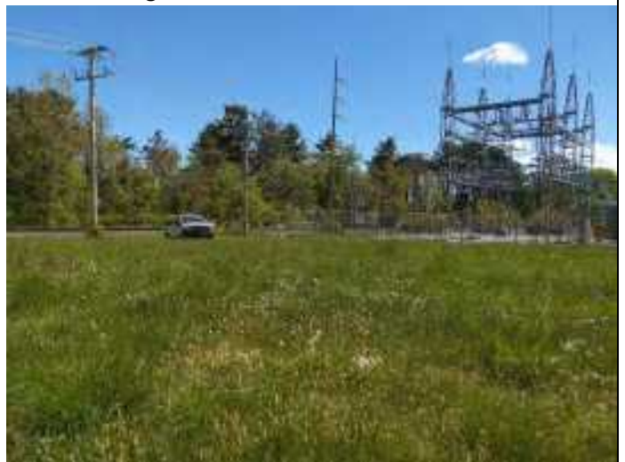
Overview of substation area near UDP-A (facing Northeast)
